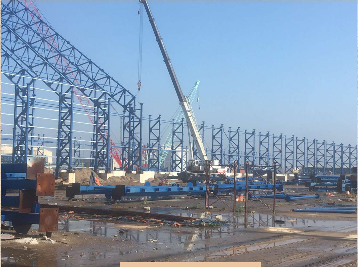
INSTALL THE COAL WAREHOUSE
